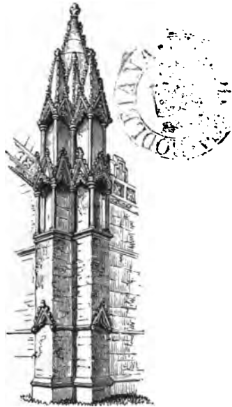
147. Gadsby, Leicestershire, c. 1350. Corner buttress with canopies and pinnacle.
